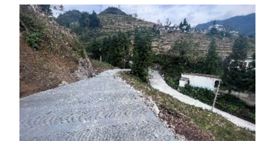
Picture: Road widening and renovation project
