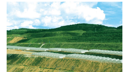
Picture: Aerial photography of reclaimed vegetation area of Kunyang Phosphate Mine
