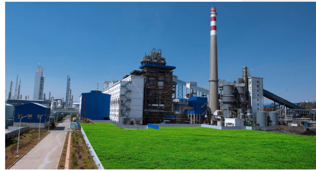
Picture above: The ammonia synthesis plant of Tian'an Chemical
